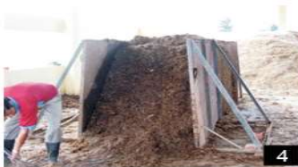
Making of Pile
