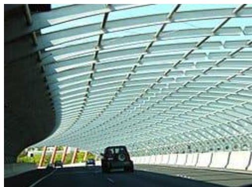
The sound tube in Melbourne, Australia is designed to reduce roadway noise without detracting from the area’s aesthetics.
